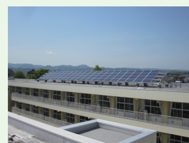
Solar panel installation subsidized by the government
