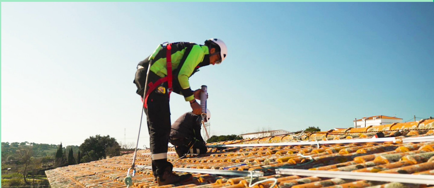
Urban solar farm in Cedillo solar village.
