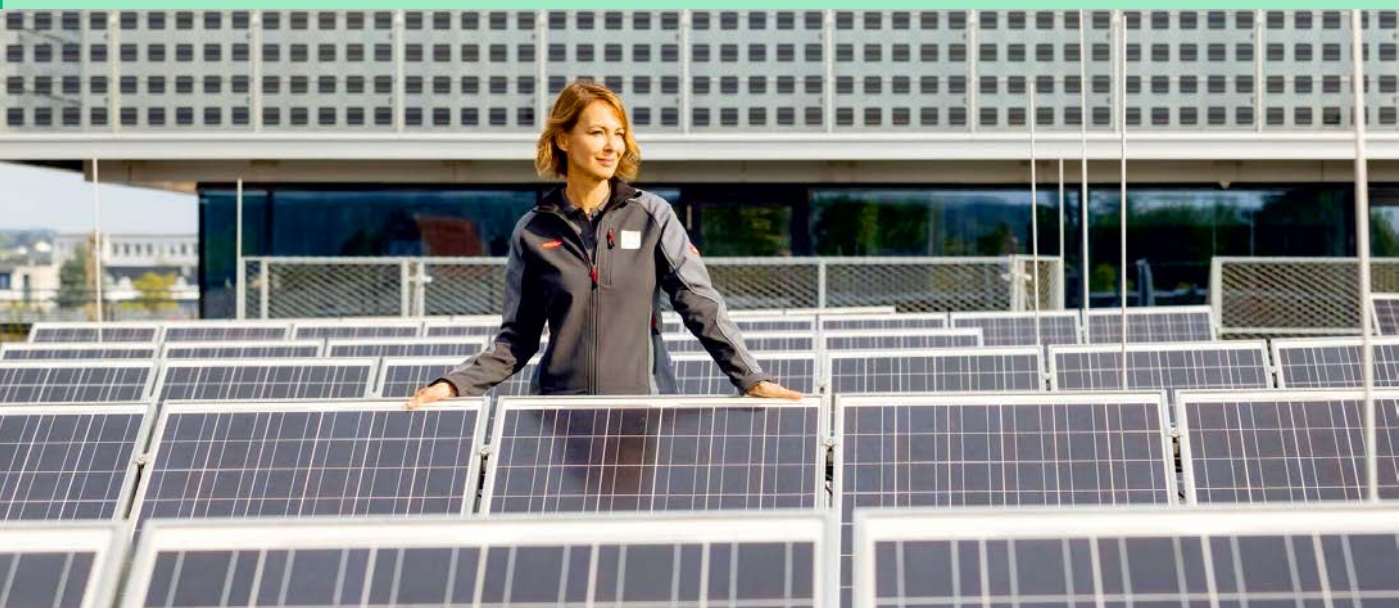
PV on the rooftop of the Fronius office in Wels, Austria.
