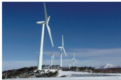
Support for the introduction of renewable energy
