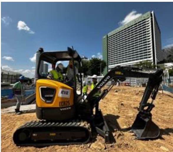
Volvo ECR25 electric compact excavator deployed at NS Square
