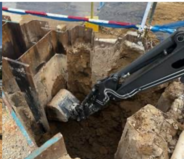
Volvo ECR25 being used to clean sheet piles at NS Square
